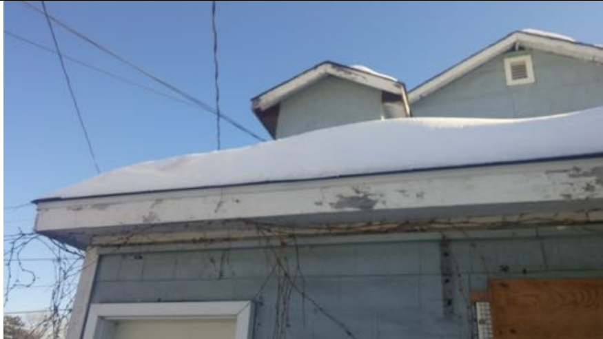
View of the flaking paint serving the fascia and soffit.
