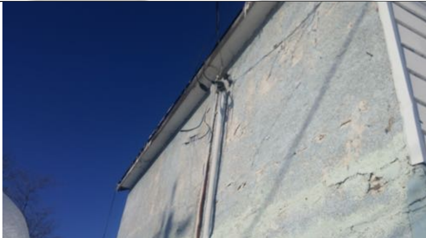
View of the missing eaves troughs serving the roof system atop the commercial building.
