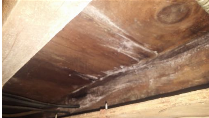
View of the typical water damaged noted within the intermediate floor system.
