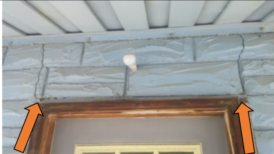
View of the missing steel lintel and step cracking above the door located on the east elevation of the commercial building.
