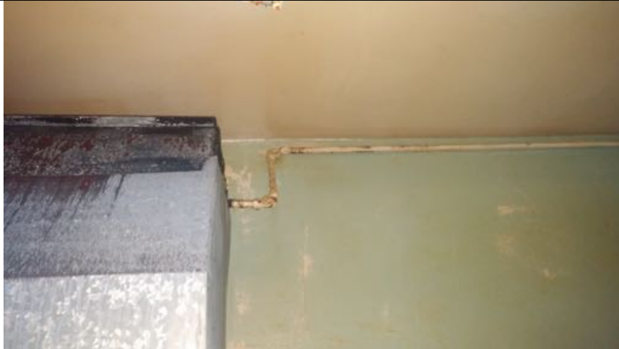
View of the typical grease and grime located in the kitchen space on the ground floor of the commercial building.
