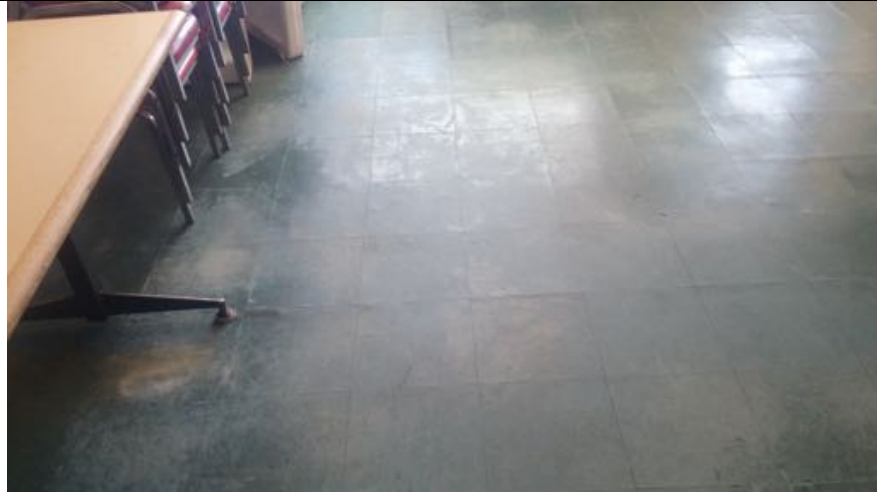
View of the deteriorating and cracked vinyl tiles serving the ground floor of the commercial building.
