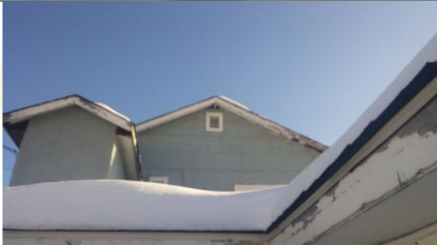
View of the gable end exhaust louvres serving the attic space atop the commercial building.
