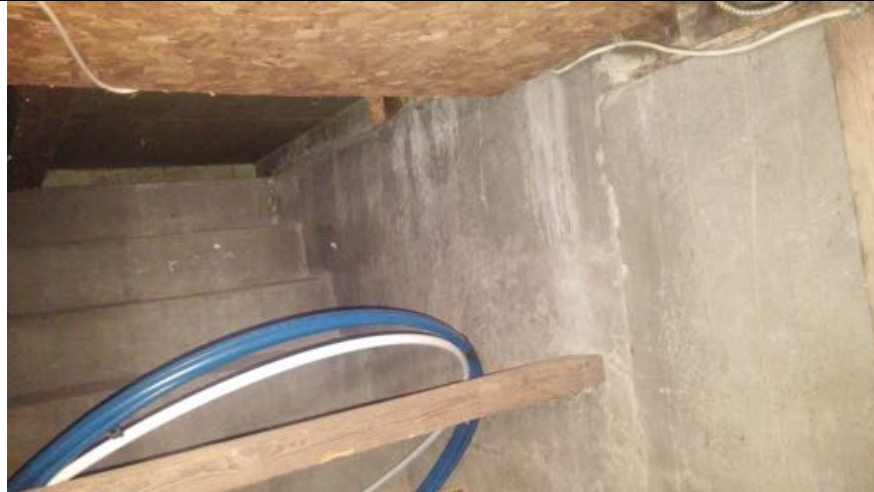
View of the typical cast-in-place concrete foundation wall serving the west portion of the commercial building.
