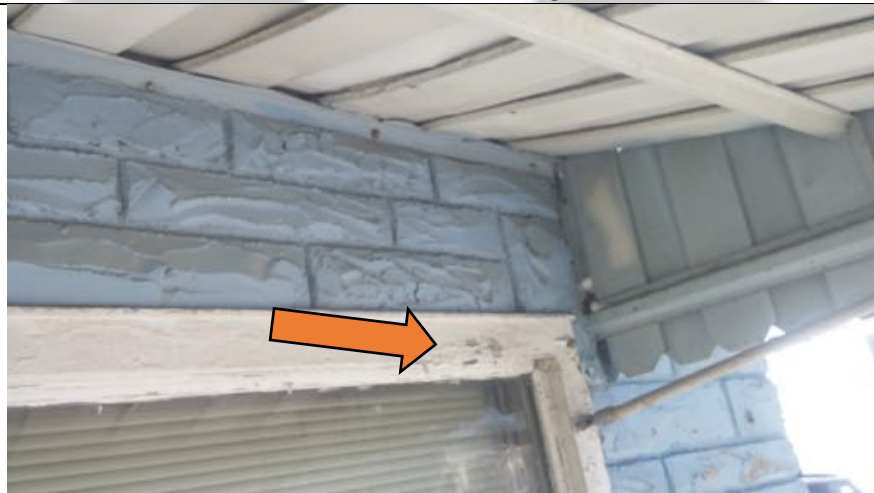
View of the flaking paint located throughout the wooden framed windows.
