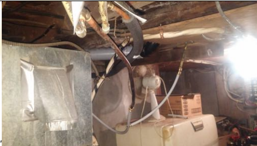
General view of the copper and cross-link polyethylene plumbing serving the supply water for the commercial building.
