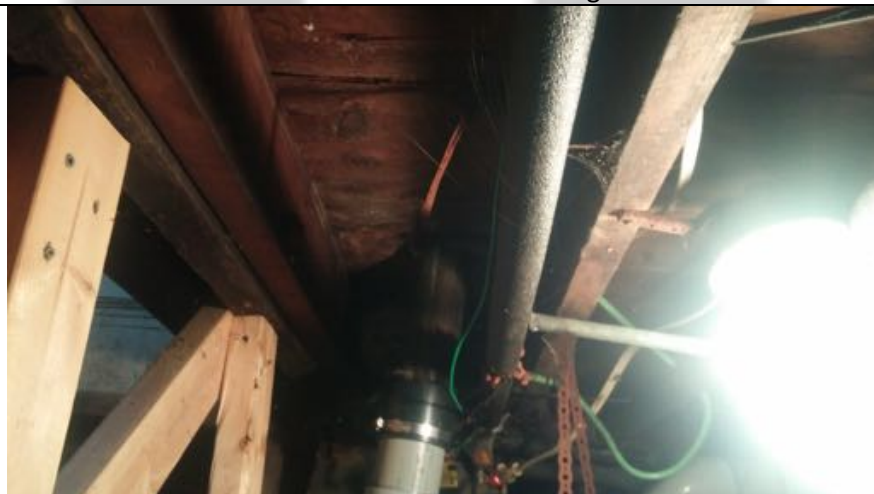
View of the typical wood framed intermediate floor system serving the commercial building.
