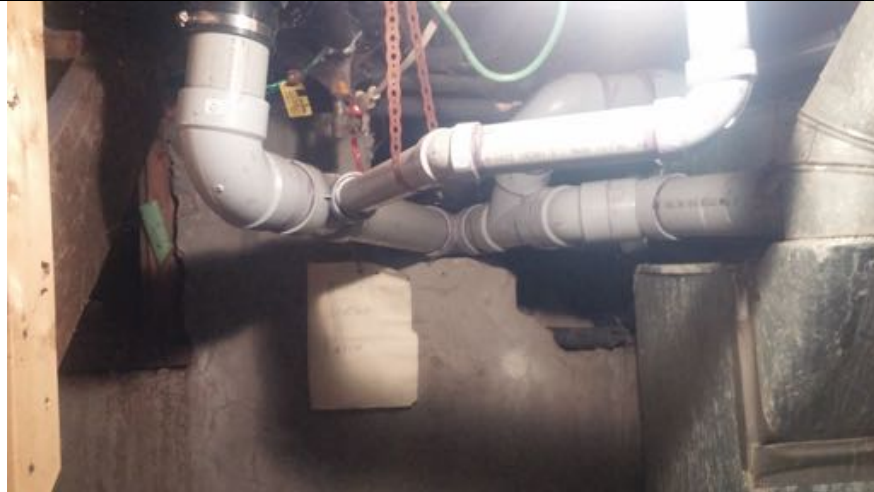
General view of the combination of ABS, cast-iron and copper sanitary plumbing system serving the residence.
