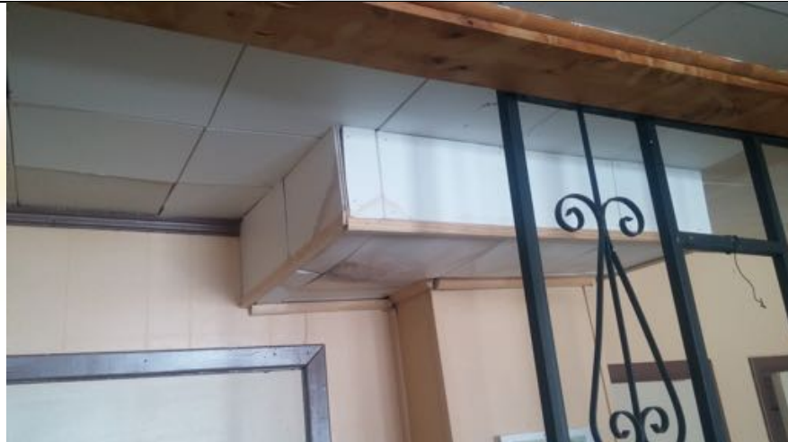
View of the typical water impacted ceiling within the ground floor of the commercial building.
