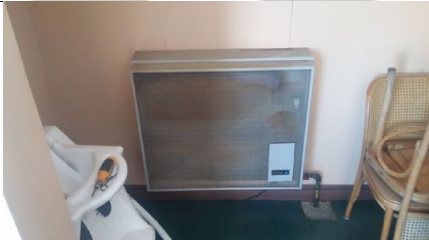
General view of the natural gas-fired "Hiunter" space heater serving the commercial building.
