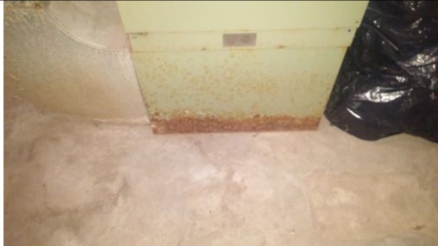
View of the corroding metal housing serving the furnace unit.
