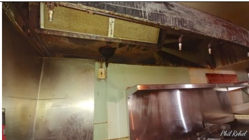
View of the wet sprinkler system serving the exhaust hood vent within the kitchen space.
