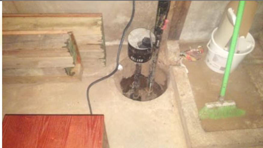
General view of the column sump pump serving the property.
