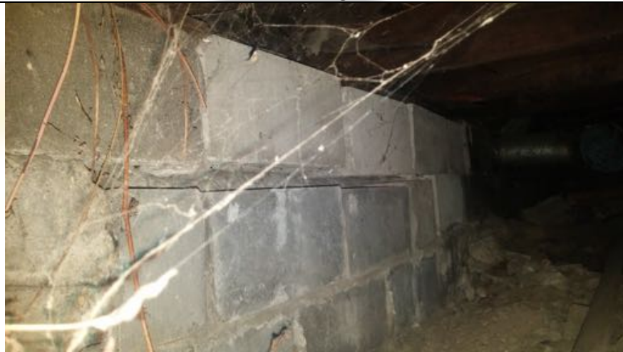
View of typical dislodged concrete block masonry perimeter foundation walls serving the east portion of the commercial building.
