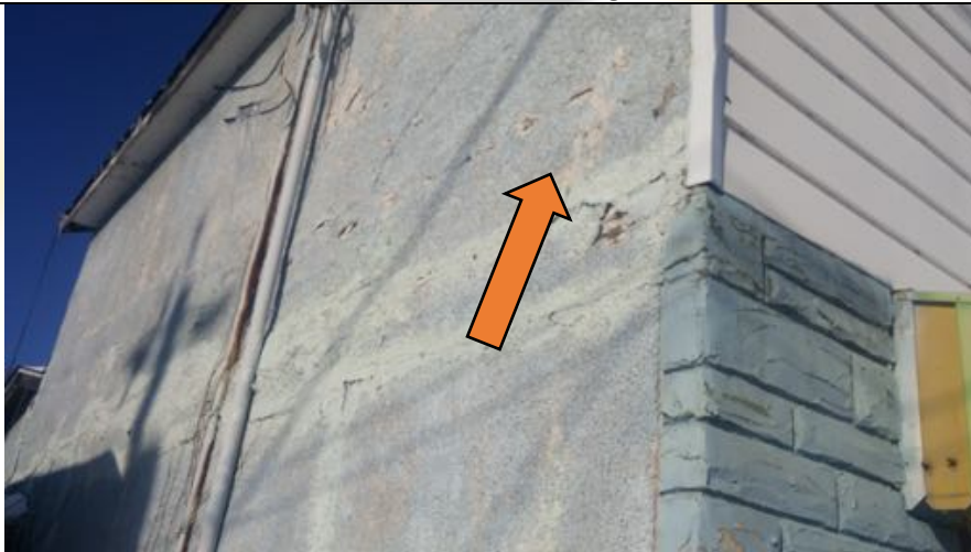
View of the typical deterioration the aggregate stucco located on the south elevation of the commercial building.
