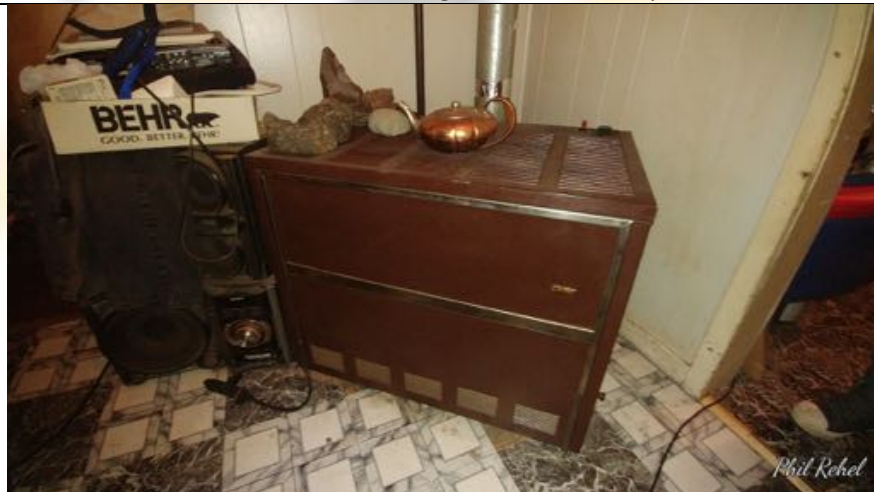
General view of the natural gas-fired "Louisville" space heater serving the residential building.
